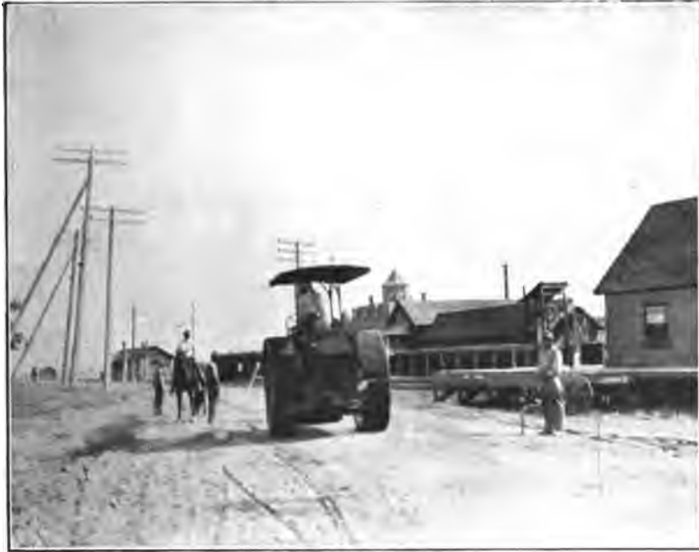
Convicts Constructing Macadam Road at Hot Springs, Box Elder County.
